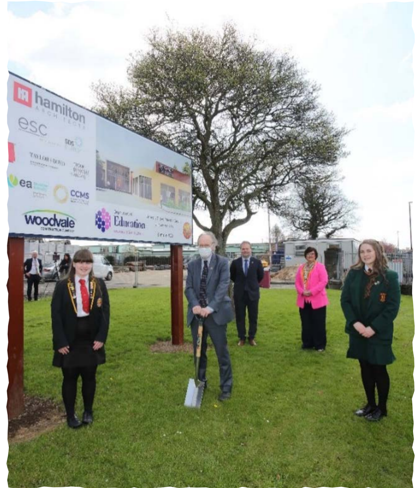
Education Minister, Peter Weir, cuts the first sod at the new Shared Education Campus site in Limavady
