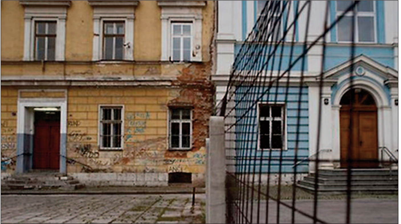
A school building in the town of Travnik in central Bosnia with a fence in between. The building hosts a primary school and grammar school for Croats/Catholics, while the yellow part of building is the secondary school for Bosniaks
